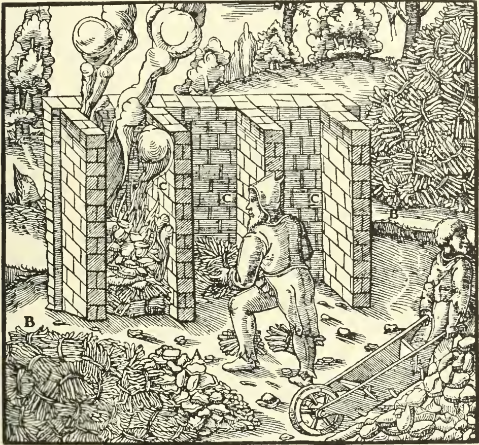
A—CAKES. B—BUNDLES OF FAGGOTS. C—FURNACES.
